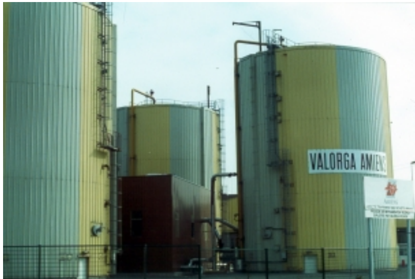
This MSW digester has operated continuously since 1988 (photo credit: Krijn Braber, NOVEM)
