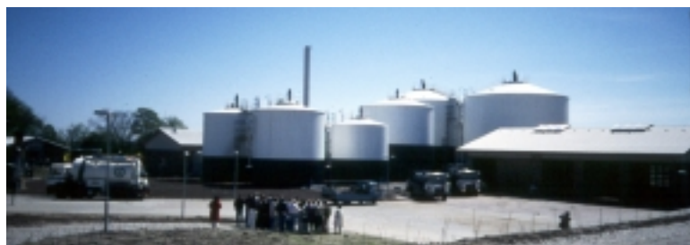
A centralized Danish digester processing manure, organic industrial residue, and biowaste
