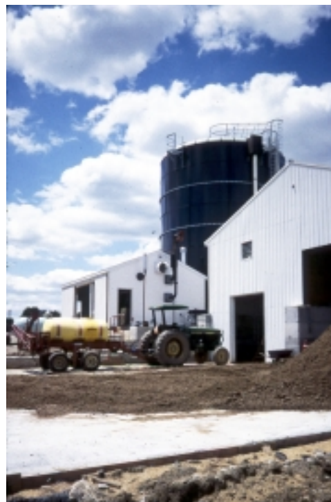
A modern dairy farm complete-mix digester that also recovers valuable fiber
